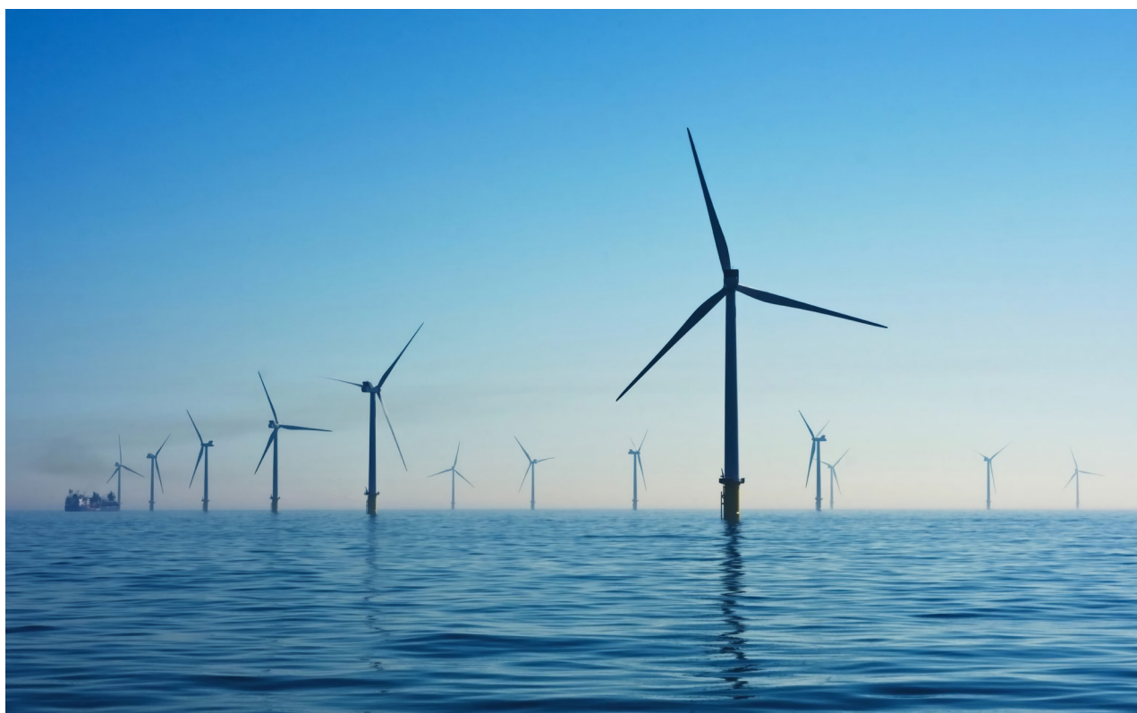
Figure 9. Rampion Offshore Wind Farm, United Kingdom
